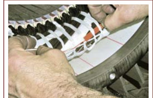
Sensor with silicone rubber body pictured above inserted near EndTurn of windings.
